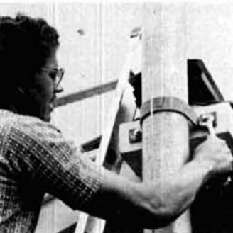
Mounting the House Bracket
