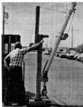
Tilting the tower over is a one-man task with the Wilson bases. (Shown above is the RB-61A.)
